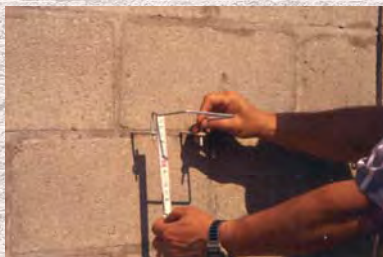
Figure 9.10 Metal ties for cavity wall construction.
