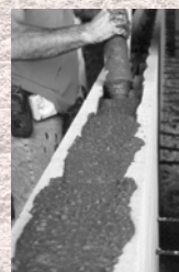
Grouting of a concrete masonry wall.
