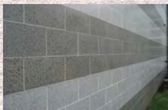
Figure 4.10 Running bond masonry.
