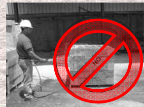
Figure 4.3 Concrete masonry units should normally not be wetted.
