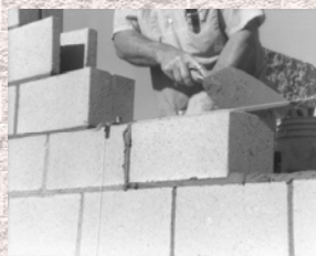
Figure 4.35 Racked masonry.
