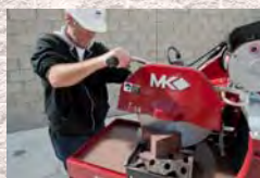
Figure 4.12 Cutting masonry units.
