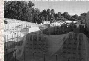
Figure 4.1 Proper storage of masonry units.
