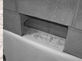
Figure 6.5 Bond beam used on first course for cleanouts.
